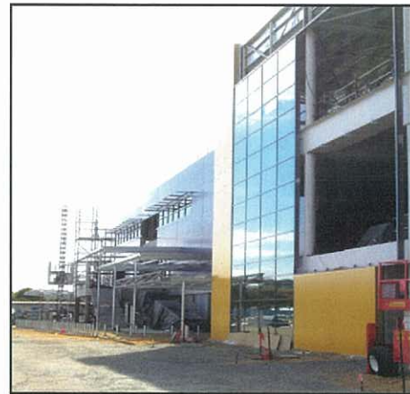
IKEA Store main entry façade under construction, October 2007
