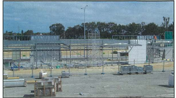
Perimeter Building # 1 under construction, September 2007
