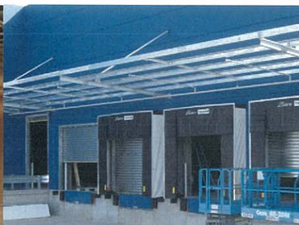
IKEA Loading Dock area nearing completion, October 2007
