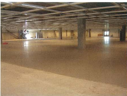
IKEA Market Hall just prior to handover, October 2007
